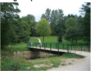
The repair to the new bridge which had taken considerable time in the planning was finally finished this Spring together with works to the river bank to prevent further erosion damaging its supports in the future.
