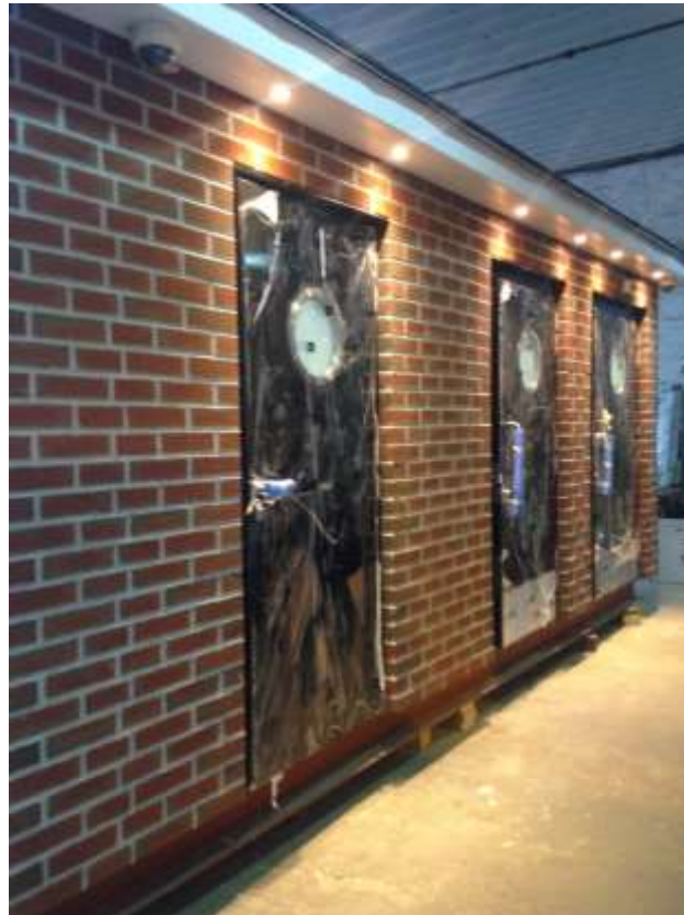
This shows the entrances to the two toilet cubicles and the refreshment facility and will face Cliff Road
